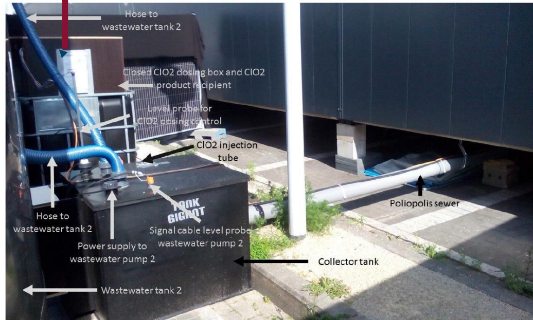
Fig. 1: Iwaki dosing pump and digital timer, situated in a locked box on the liquid chlorine dioxide product recipient.
