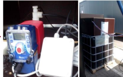
Fig. 1: Iwaki dosing pump and digital timer, situated in a locked box on the liquid chlorine dioxide product recipient.
